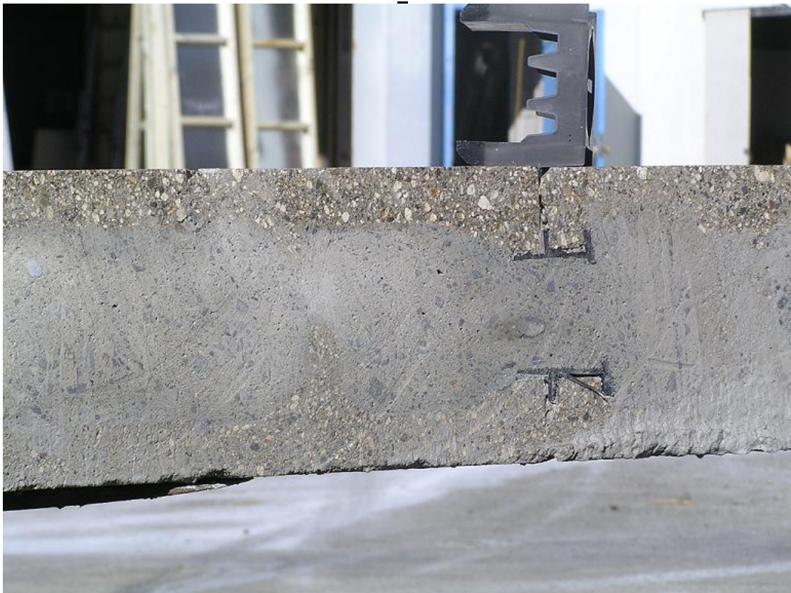
Figure 2 – Close up of cut wall.
