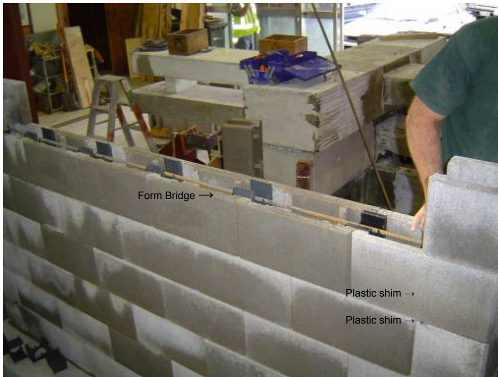
Figure 4-2 Wall construction showing Form Bridges and plastic shims
