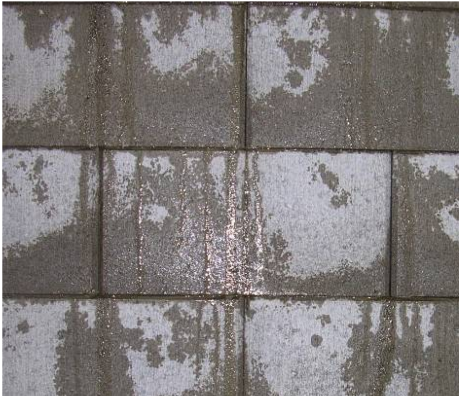
Figure 7-1 Openings in joints on wall before testing
