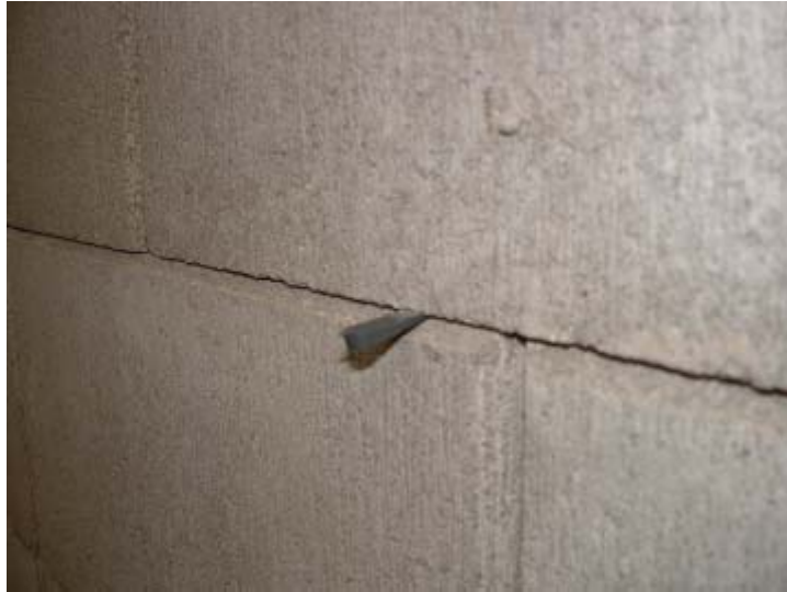
Figure 4-3 Plastic shims positioned at joints
