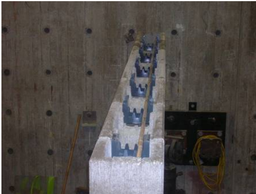
Figure 4-4 Reinforcement alignment using Form Bridge
